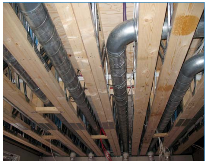
Floor Joists parallel to the external panel
